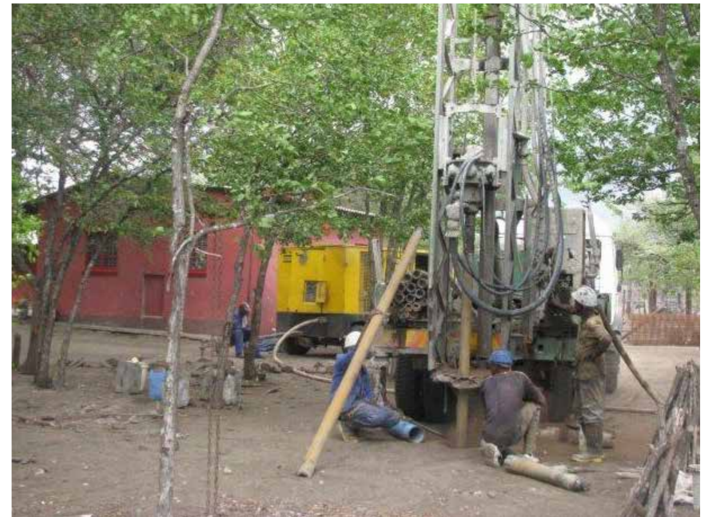
Borehole drilling in the LCV grounds
